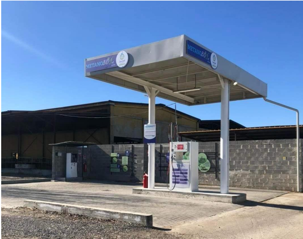
Figure 141: Public CNG refueling station Source: Agriturismo Bosco Gerolo
