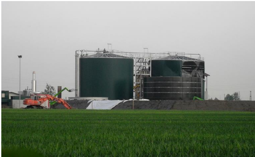
Figure 27: Biogas plant of Lendinara Source: SantafoCADelfriuli.it
