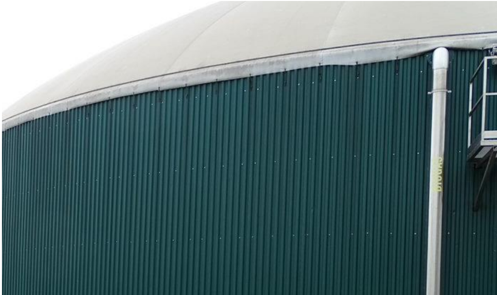
Figure 45: Gasometer-wall junction Source: Principi di Porcia e Brugnera
