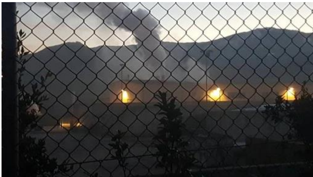
Figure 34: Biogas plant of Acqualagna Source: Ilrestodelcarlino.it
