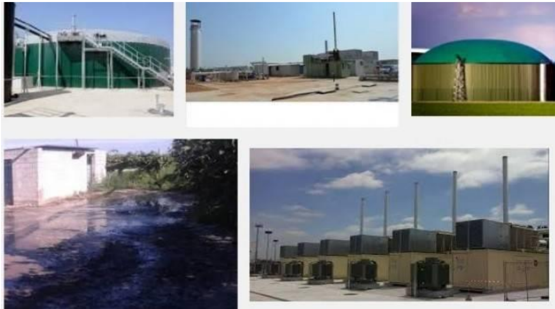
Figure 32: Biogas plant of Roverbella (MN) Source: Sgonfiailbiogas.it
