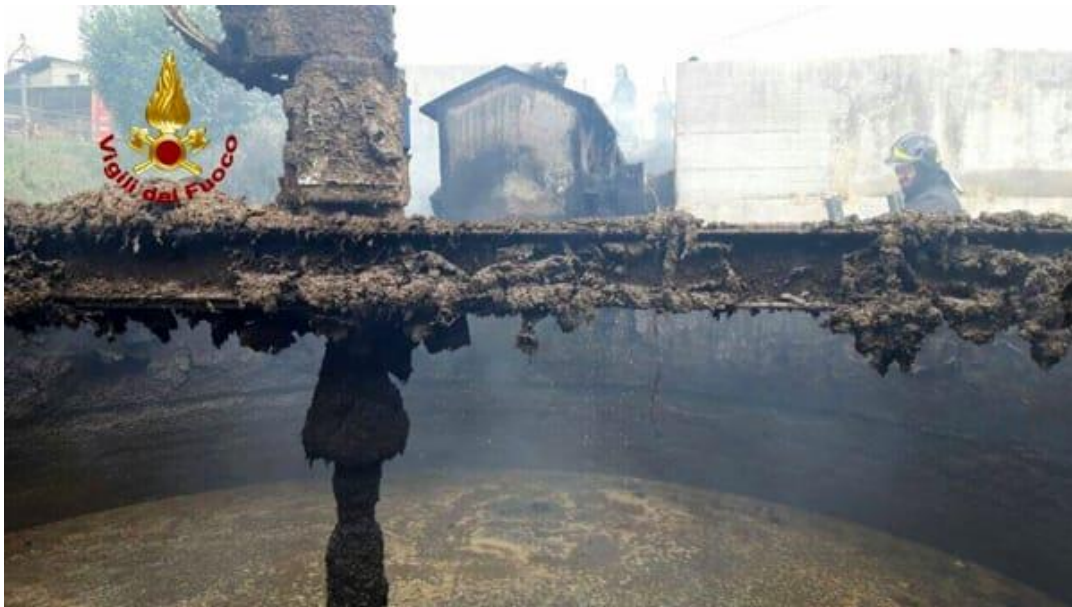
Figure 30: Biogas plant of S.Egidio (PG) Source: Corrieredellumbria.it
