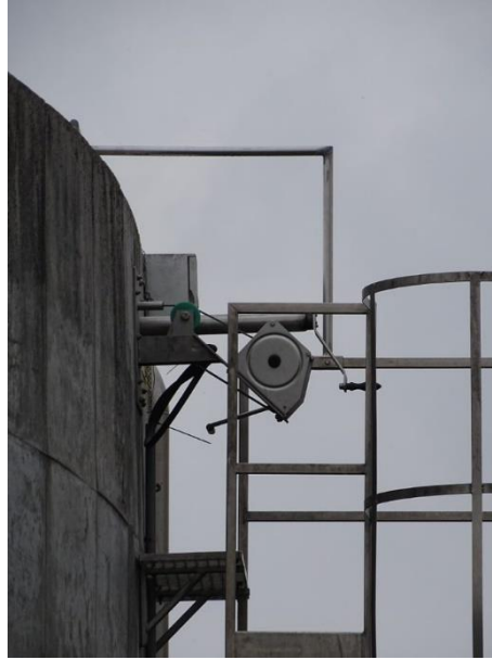
Figure 41: Winch for mixer height variation Source: Principi di Porcia e Brugnera
