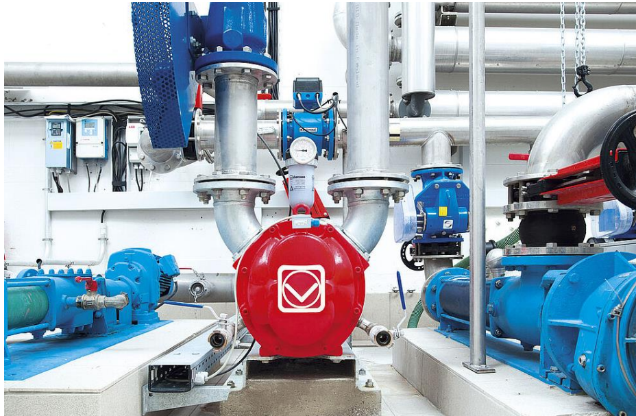
Figure 16: Lobe pump for slurry Source: Vogelsang
